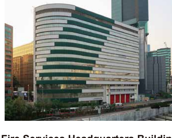
Fire Services Headquarters Building
