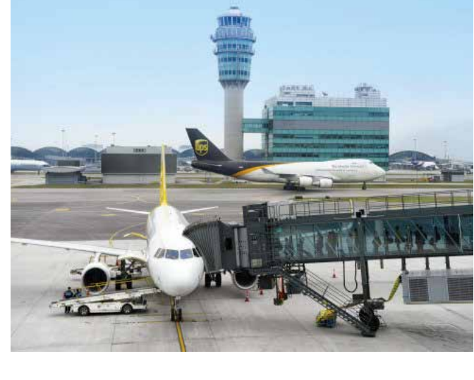
Hong Kong International Airport
