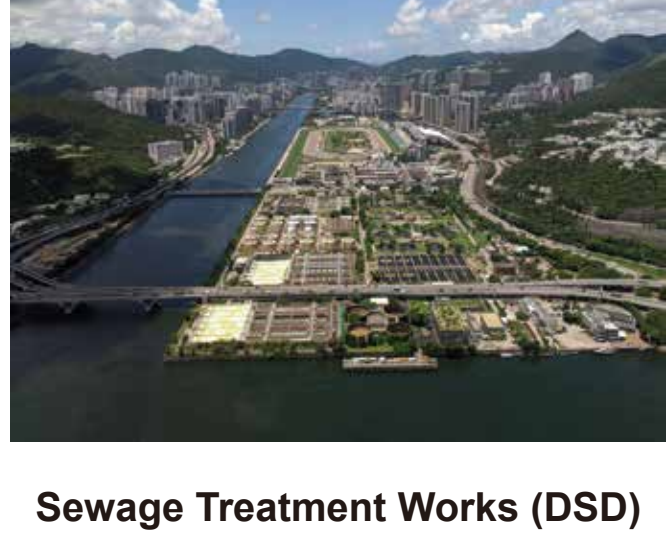
Sewage Treatment Works (DSD)
