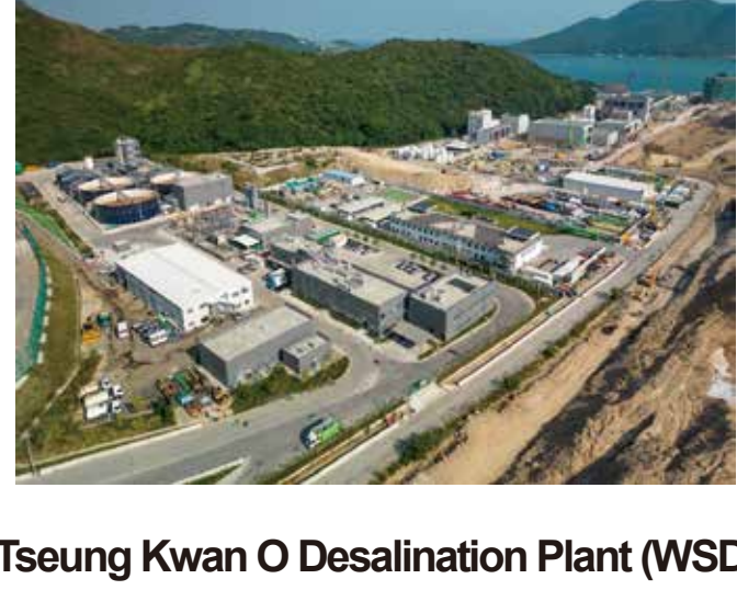
Tseung Kwan O Desalination Plant (WSD)
