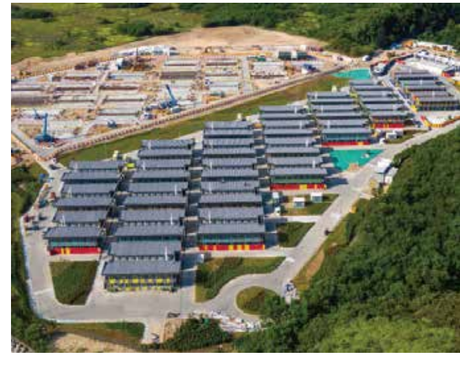
Temporary Quarantine Centre at Penny's Bay
